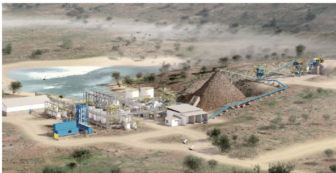
Turnkey gold ore processing plant with a production capacity of 35 tph / Ethiopia
