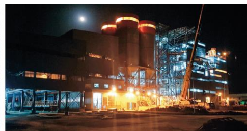
Turnkey cement grinding plant with a production capacity of 135 tph, ball mill (inside Ø: 4.6 m, length: 15 m, drive power: 4.700 KW) / Ghana
